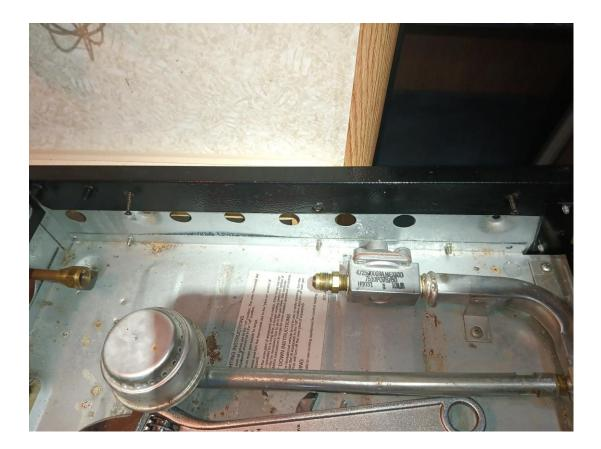
Turn on the propane and test for leaks using soapy water near the threads or better yet put your nose right to the fitting and smell. If gas is detected then more than likely the fitting requires tightening. If no gas is detected continue on.
