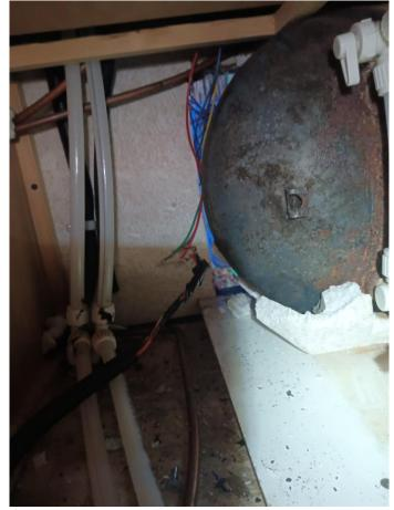
Remove the bypass valves PEX tube in order to remove the valves from the tank. The PEX will need to be heated in the middle and on one end to facilitate removal.
